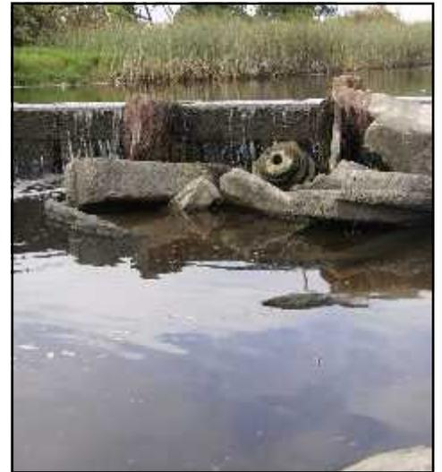
*The weir at the mouth of the lagoon currently prevents ocean tides from entering to clean, cool, and add oxygen to the lagoon's water. If the weir were removed, the open channel would also allow silt and sand to be flushed from the lagoon, and provide an avenue for fish and other marine organisms to follow their natural instincts and needs to freely move between the ocean and the lagoon.*
